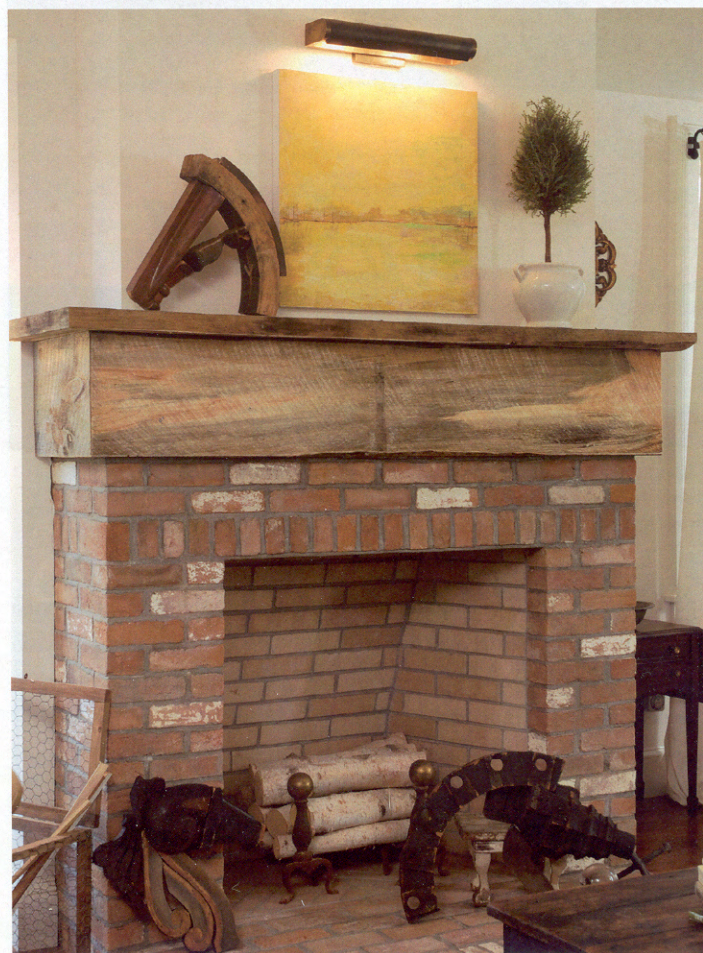
Original bricks from the home were used as part of the new fireplace. Bill Muscara constructed a mantel with rough-sawn lumber, which mirrors the materials and techniques that were employed almost two centuries ago.
